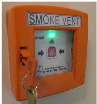
4. The green light will show if all OK. The middle red one ONLY needs pressing to actually open the windows, done monthly checks. Press the right button with the down arrow to re-set.
