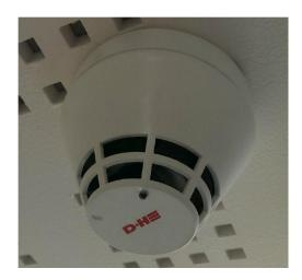
2. Unscrew the top off this detector, blow into the piece that has come off, and re-screw back on.
